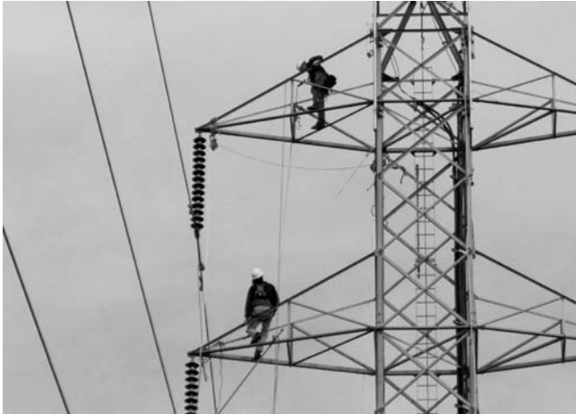
FIGURE 1.4 A transmission line that is being upgraded.
