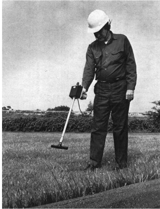
FIGURE 5.44 Lightweight battery-operated cable route tracer. (Courtesy of James G. Biddle Company.)
