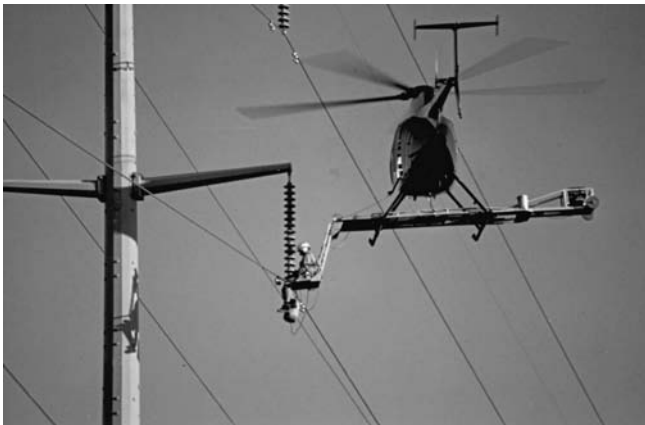
FIGURE 2.15 A lineman working from a helicopter platform.
